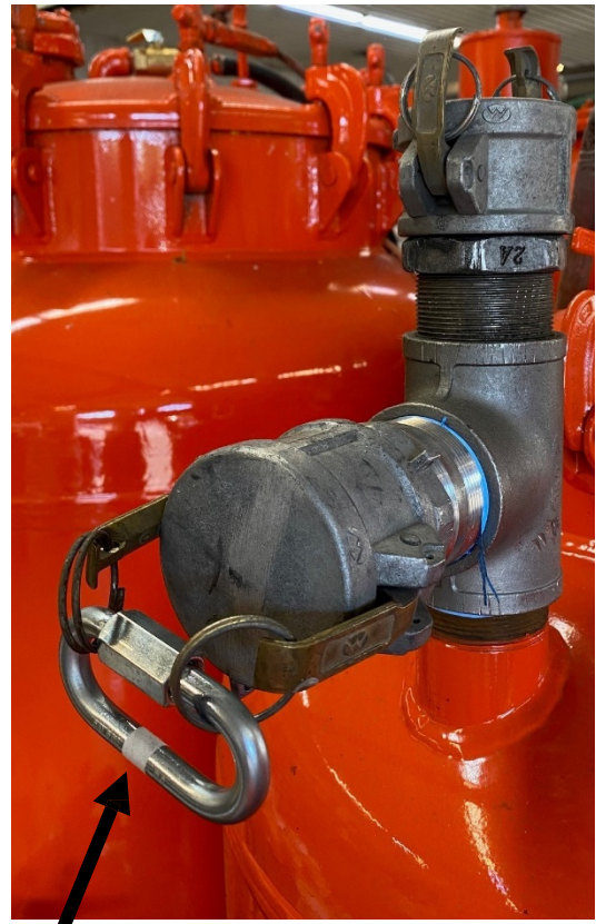
Oval Threaded Link securing the cam-locks
